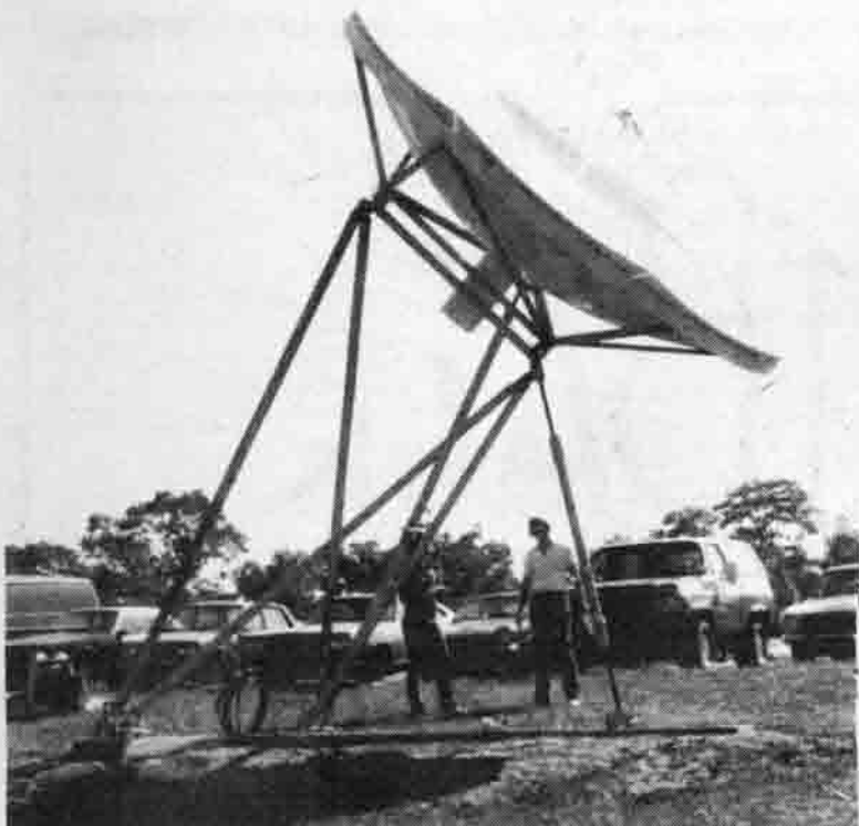
SPACE-AGE SIGHT: UMSL radio station KWMU will use this satellite dish installed east of Clark Hall to pick up a 24-channel supply of constant programming from the orbiting WESTAR I [photo by Wiley Price].
